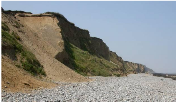
Fig. 5: West Runton, looking west of the slipway.
