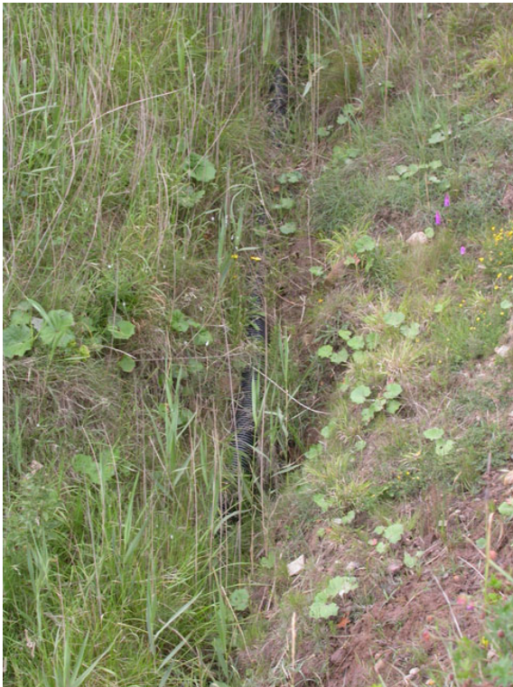
Fig. 5: This seepage should be restored by removing the drainage pipe. Seepages at Blackhall Rocks are important for invertebrates but at least one has been diverted into a section of plastic pipe (Fig. 5). This should be removed as soon as possible to allow natural drainage.
